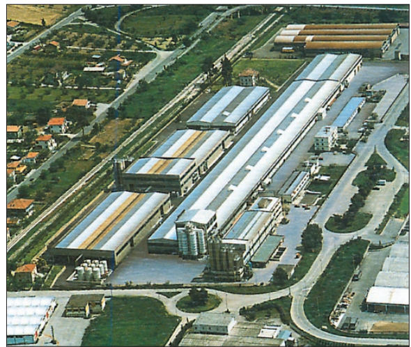
Alfagomma Rubber Industrial Hose Manufacturing facility-Teramo, Italy
