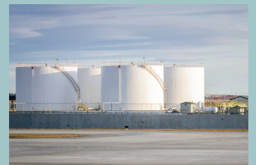
Tank to Tank
