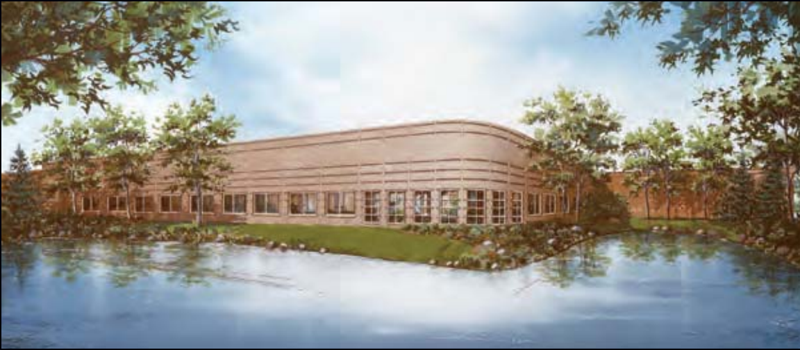
Vernon Hills, Illinois: Headquarters/Plant
